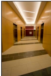
Modern Tile & Stone of Dallas collaborated with Dee Brown on this project. Following the pattern of light and brown stone, Clint Bunch and his crew from MTS placed smaller versions of the limestone at the same 20-degree angle in the elevator lobbies on four floors of the building. They also used *Ultracontact RS* and *Keracolor U* for these installations. Inside the elevator cabs, they installed the stone with *Granirapid* mortar and grouted with *Keracolor U*.
