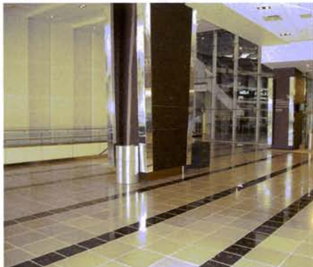
Modern Tile installers' work highlights straight, even grout lines. Courtesy of Modern Tile Co., Inc.
